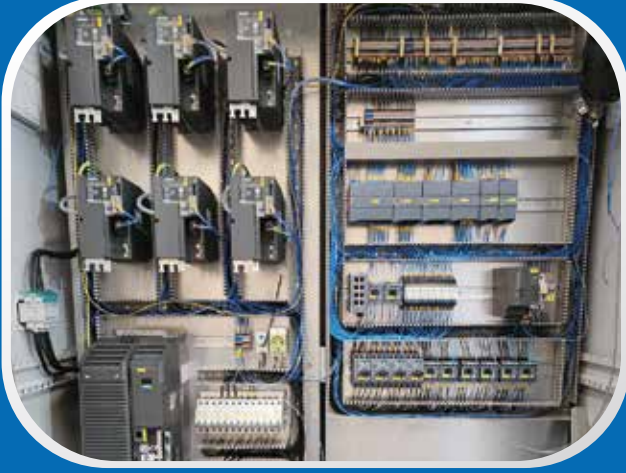
Siemens Elektrik Panosu Electric Cabinet with Siemens Components
